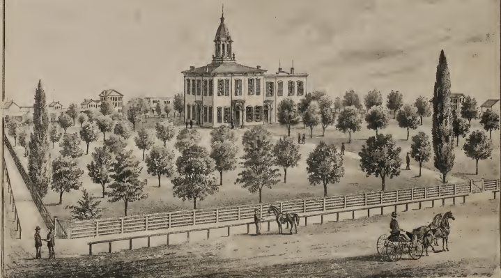
HANCOCK COUNTY COURT HOUSE, CARTHAGE, ILL.
